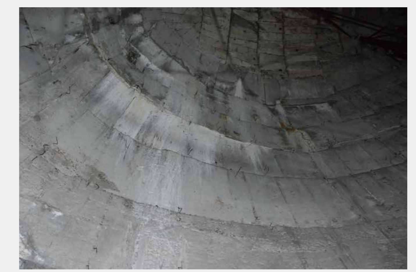
Traces of the formwork that remain inside the Great Buddha
